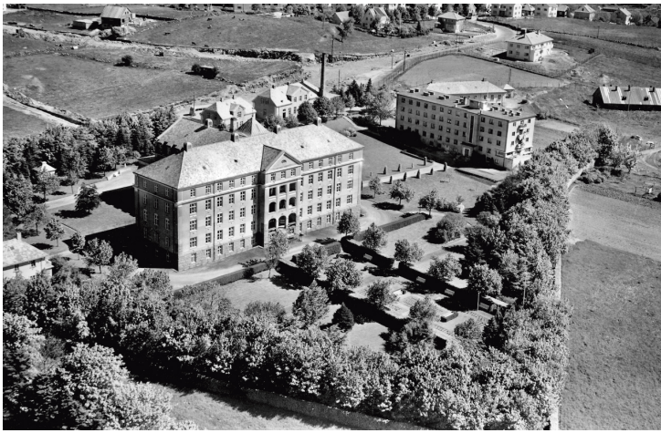
Figure 3 Rogaland Hospital photographed in 1951 by Widerøe Flyselskap [Widerøe Airlines]. The building to the right of the hospital is the Red Cross Nursing School. The white house on the right-hand side of the photograph is the old senior consultant accommodation. Photograph reproduced with the permission of Stavanger City Archives.
