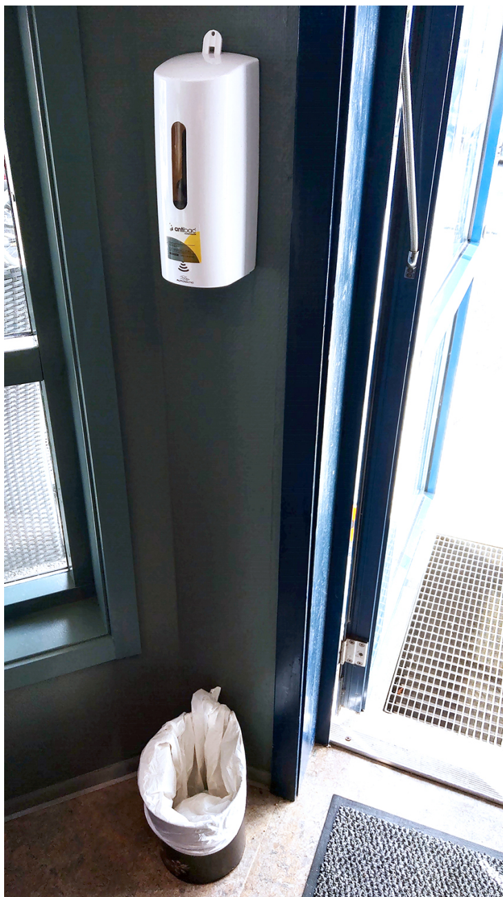
Waste bins placed directly under alcohol-based disinfectant. Photo: Arnstein Fedøy
